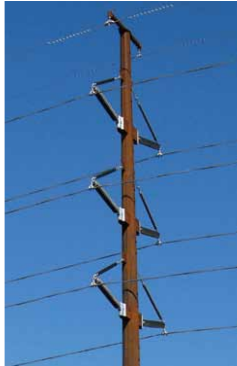
Weathered-steel poles will be used along most of the route.
