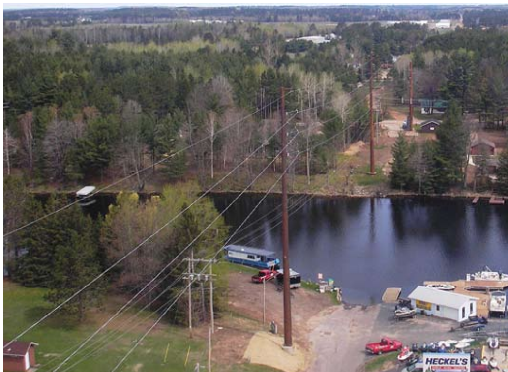
Some of the tallest poles on the project – 115 feet – were used to cross the Eagle River.
