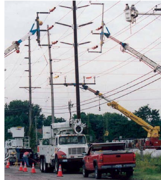
On a similar project, workers string wires on the structures.
