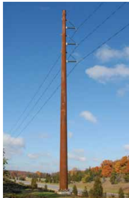
Weathering steel poles, which appear brown in color, will be used for the majority of the 18-mile line.
